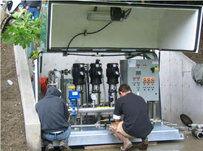
frequency drives. In addition to pump control, the custom control panel includes controls for the storage tank, the upstream chlorinator and automatic switching during "tank bypass" operation.
