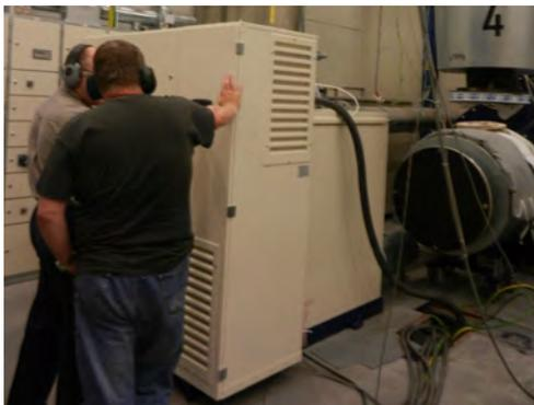
One of the key selection criteria was the oil free magnetic bearings used in these blowers. The magnetic bearings keep the motor rotor shaft levitating
