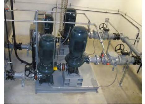
gpm at 350' TDH. Airvac worked with L2 Systems in Everett to assure that local support would be available for all of the controls. The control system was designed to provide both reliability and redundancy complete with spare pumps & VFD's.
