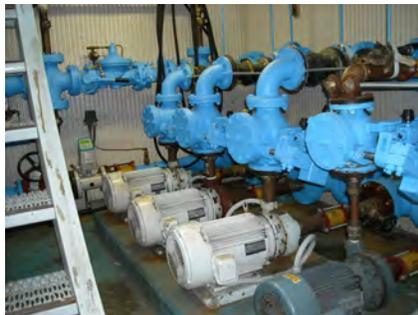
utilized four 3HP vertical multistage pumps controlled by variable frequency drives (VFD's). These new duty pumps are inherently more efficient as well as more energy efficient due to the variable frequency operation. Electrical savings have averaged 38.4% over the past seven months.
