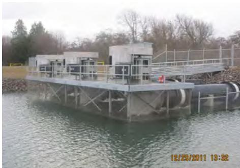
from Watts Constructors for the 3 pumps. Each 300 HP pump is capable of pumping 69,700 gallons of water per minute from the flooded area
