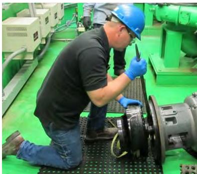
This test pump was installed in a underground, dry pit station manufactured by Dakota Pump and supplied by PumpTech. It had a history of ragging due to the make up of the wastewater entering the pump station. Since the retro-fit, it has not experienced any ragging or plugging and the pump operates at its design point. In the past ten years, ragging has become more of an
